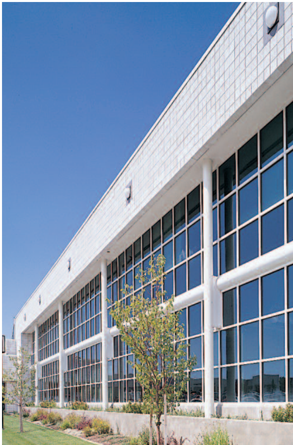
St. Benedict's Medical Arts Building, Ogden, UT Architect: Babcock Design Group
